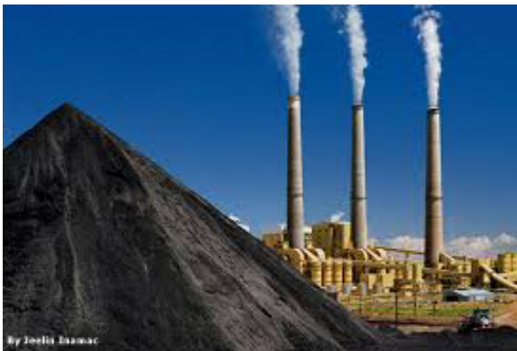
Figure 1 - A Coal-Fired Power Plant
