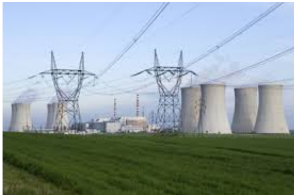
Figure 5 - A Nuclear Power Plant with Water-Cooling Towers and the Beginning of the Electrical Grid in the Area.
