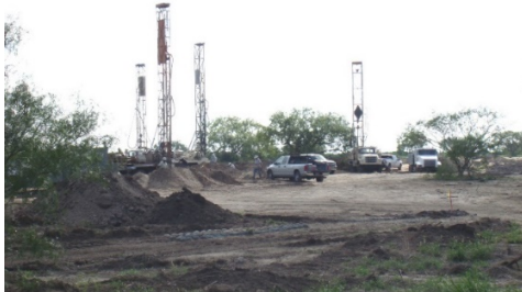
Production Drilling in South Texas
