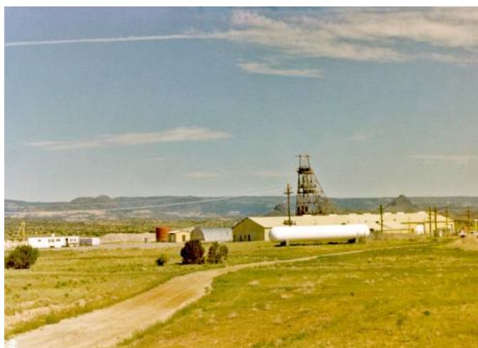
Figure 10. Surface plant at Kermac's Rio Puerco mine, Sandoval County. Photo by W.L. Chenoweth in 1981.
