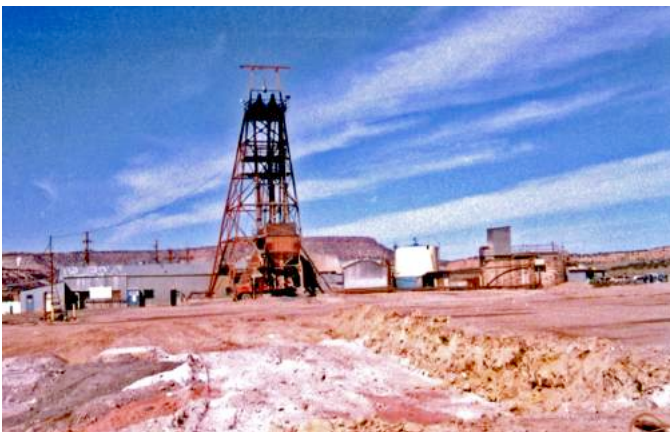
Figure 3. Surface plant of Kermac's Section 22 mine, Ambrosia Lake subdistrict, McKinley County. The headframe is for a shaft that is 826 ft deep. Photo by W.L. Chenoweth in 1961.
