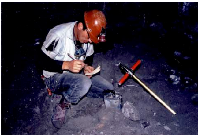
Figure 5. Grade control engineer checking grade of blasted ore with a T-probe at the Homestake-Sapin Partners Section 25 mine, Ambrosia Lake subdistrict, McKinley County. Photo by U.S. Atomic Energy Commission geologists in the 1960s.
