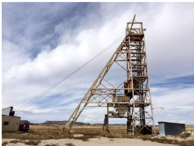
Figure 14. The eastern headframe of the Section 11/12 mine, Ambrosia Lake sub-district, McKinley County. The mine shaft is 500–520 feet deep (George Lotspeich, Hydro Resources, personal comm., 2014). Cumulative production from 1961–1963 was 211,873 pounds U_3O_8 , with a production grade of 0.15% U_3O_8 , likely depleting the deposit resource. The mine operated until 1980 (McLemore et al., 2013). Photo by Bonnie A. Frey in October 2014.
