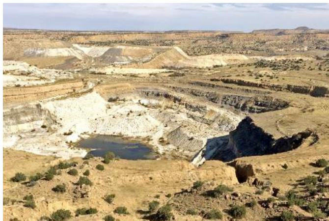
Figure 17. St. Anthony mine west pit viewed from the west–southwest. Waste piles are visible behind the pit. The cumulative production of the mine from 1953–1960 was 2.5 million pounds of U_3O_8 with a production grade of 0.17% U_3O_8 . Vanadium was also recovered. The historic resource estimate was about 3.9 million tons of ore (McLemore et al., 2013). Photo by Bonnie A. Frey in October 2015.
