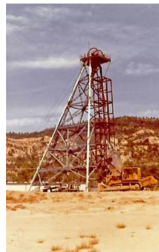
Figure 9. Bokum Resources shaft at Marquez Canyon, McKinley County. Shaft was never completed due to high water flow. Photo by W.L. Chenoweth in 1981.
