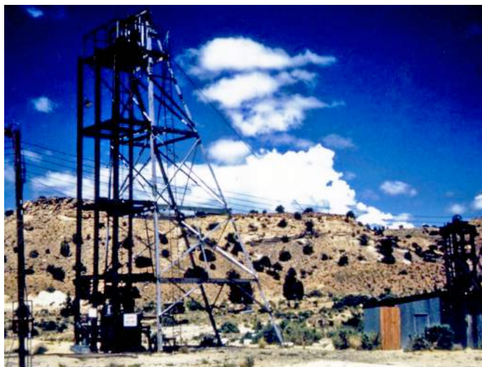
Figure 8. Headframe of Anaconda's Woodrow mine, Laguna subdistrict, Cibola County. The 230 ft deep shaft was adjacent to a collapsed ore-bearing breccia pipe in the Jackpile and Brushy Basin members of the Morrison Formation. This mine produced 5,326 tons of ore averaging 1.26% U_3O_8 , 1953–1956. Photo by W.L. Chenoweth in 1961.
