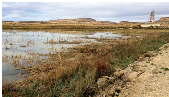
Figure 13. Ambrosia Lake in a rare moment when the lake contained water, October 2014. The structure in the background is the Section 12 headframe of the Section 11/12 mine, owned by Hydro Resources. The mine has a second headframe at the west end of the mine, in Section 11. Photo by Bonnie A. Frey.
